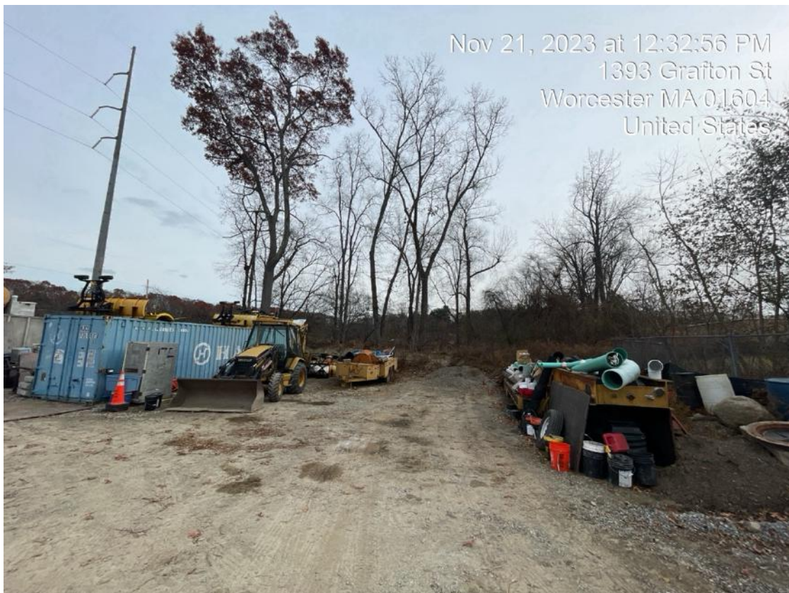
Photo 1: View of the 0 McAvey Way parcel facing southeast. BVW is located beyond berm in background of photo.
